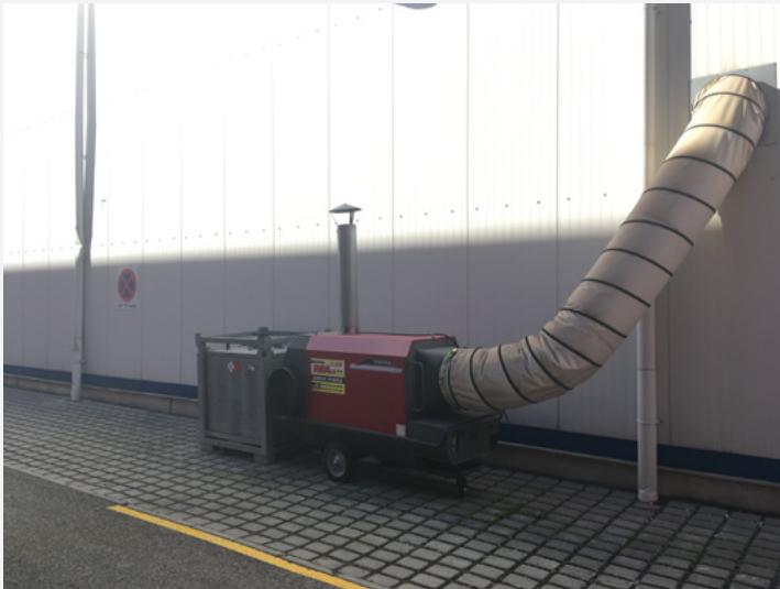
OIL HEATING SYSTEM
